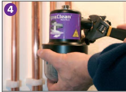
4 Loosely secure the *MagnaClean TwinTech* canister to the valves, following the flow direction indicated on the canister. Tighten the compression fittings, being careful not to over tighten.
