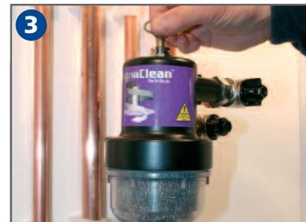
3 Replace the Pro-Fill air vent. Allow the system to circulate for 30 seconds. Open the Pro-Fill screw two turns and back-flush until clear.
