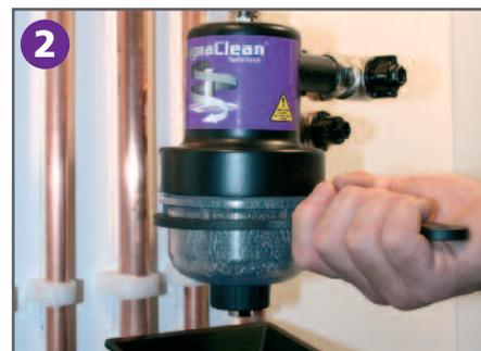
2 Loosen the canister base with the large spanner while holding the tray beneath. Carefully unscrew the clear base. Allow water to collect in the servicing tray supplied.
