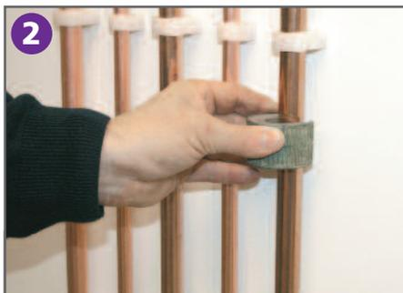
2 Using a suitable cutter, carefully remove the marked section of pipework to create the correct opening.
