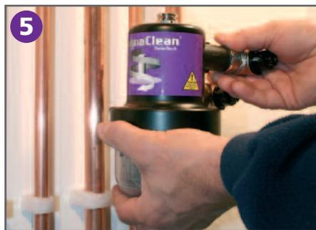
5 Loosen off the valve flange nuts and insert the rubber washers provided. Tighten the flange nuts. Do not over tighten. Refill the heating system.
