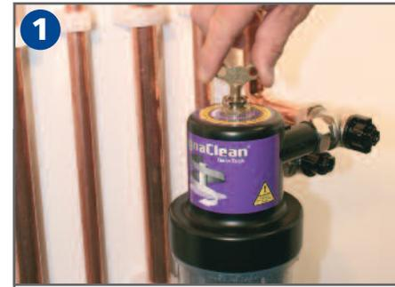
1 With a standard radiator key, remove the Pro-Fill air vent. The built-in, one-way valve will prevent water from escaping. Attach the chemical adapter and feed in the chemical.
