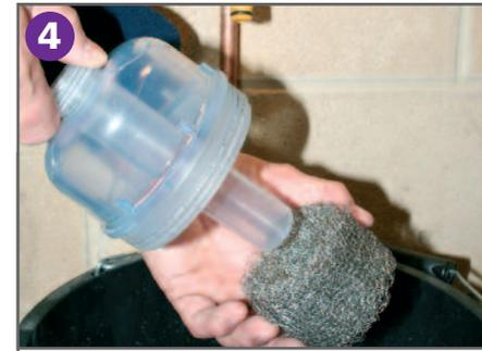
4 Remove the wire gauze and rinse. Wipe and clean out the clear base. Replace the wire gauze and the magnet cap.
