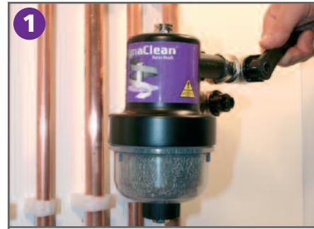
1 **Important** - Before commencing any servicing work, turn off the electrical supply to the boiler. Turn both isolation valves to the marked OFF position. Loosen the air vent to release internal pressure. When venting, protect the surface below the canister with the servicing tray provided to capture any drops of water.
