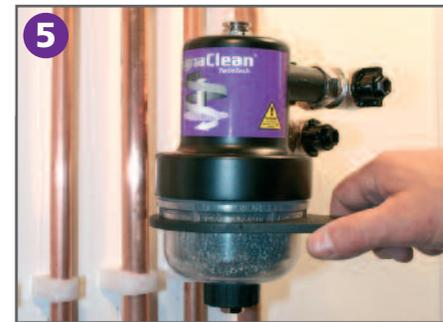
5 Re-attach the clear base to the top section of *MagnaClean TwinTech* and tighten until sealed. Do not over tighten.
