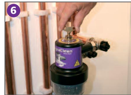
6 Open the isolation valves to the marked ON position and vent through the Pro-Fill air vent. When venting, protect the surface below the canister with the servicing tray provided to capture any drops of water. Run the central heating system while checking for leaks. Repeat steps 1 - 6 if required. Ensure the filter is thoroughly clean before leaving the premises.
