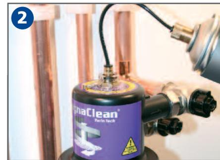
2 Wait five seconds before removing the adaptor. The Pro-Fill air vent will accept all market-leading chemicals in either liquid or concentrate form.
